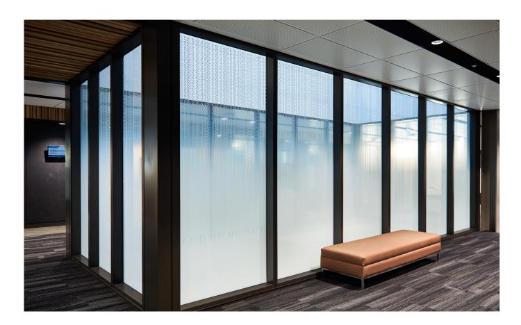
SWITCHABLE GLASS IS A LAMINATED GLASS WITH A LIQUID CRYSTAL INTER-LAYER THAT CARRIES AN ELECTRICAL CHARGE. WHEN CURRENT RUNS THROUGH THE GLASS INTER-LAYER THE CRYSTALS ALIGN WHICH MAKES THE **GLASS TRANSPARENT.**
