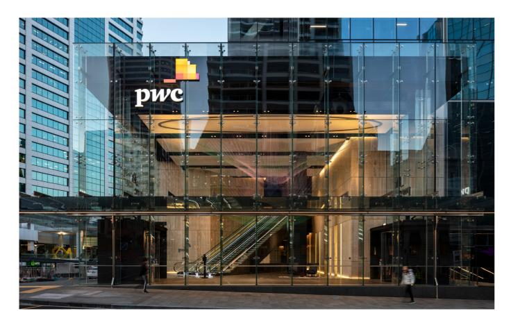
TOTALVISION IS A HIGHLY ENGINEERED FRAMELESS GLASS FACADE. THIS TOTAL VISION SYSTEM UTILISES STRUCTURAL GLASS FINS AND FITTINGS LIKE STAINLESS STEEL SPIDER FITTINGS IN ORDER TO OFFER UNENCUMBERED VIEWS AND A STUNNING AESTHETIC.
